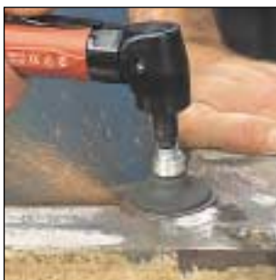
PLANING DOWN WELD
